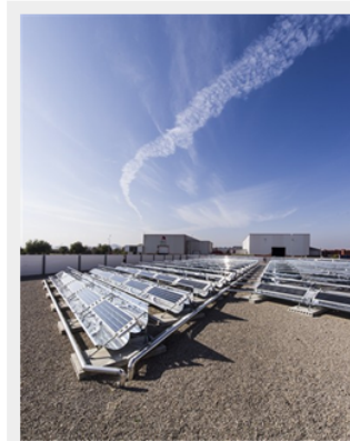
SRB Solar Panel - Solar field from Valencia
