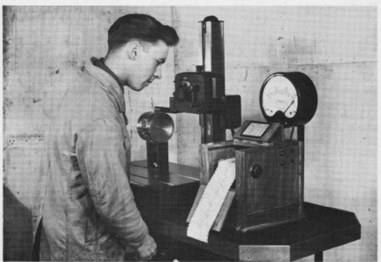
FIGURE 62 – The first Talysurf instrument
